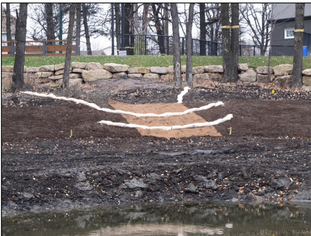
Figure 6.4. Check dam installed in upland area of an NSP, in conjunction with erosion control blanket, prior to the installation of wetland vegetation.
