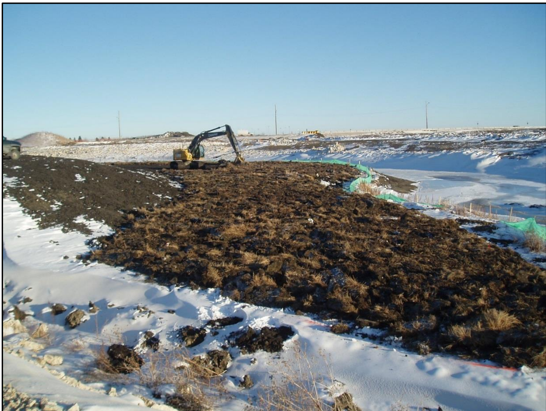
Figure 6.2. A sediment control fence at the wetland/open water interface, preventing erosion into the open water zone.
