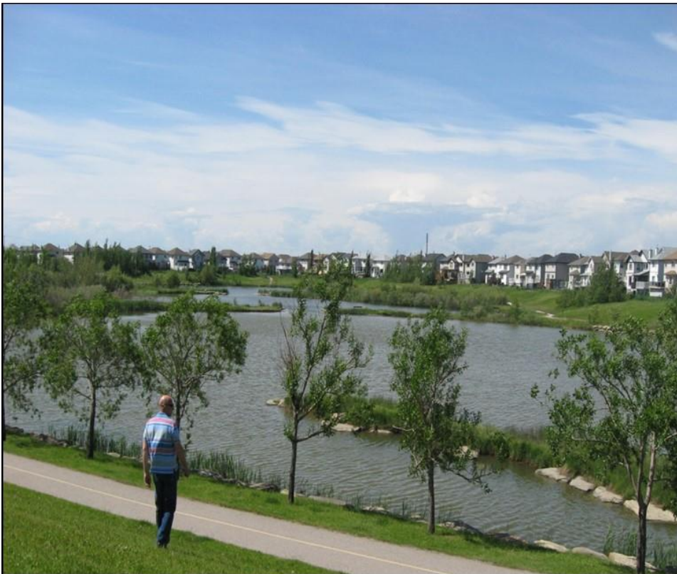
Figure 1.3. Constructed stormwater wetland in the City of Calgary, containing only a periphery of wetland vegetation.
