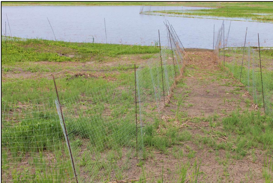
Figure 7.2. Goose deterrence fencing installed around the wetland zone of an NSP in its first commissioning year, including an entry/exit point to the open water zone from then upland area.
