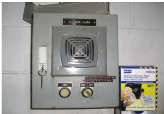
Photo 5.9: ↑ Chlorine Alarm
