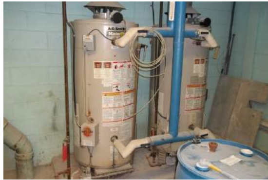
Photo 4.42: ↑ Water Heating System – Recarbonation Equipment Room
