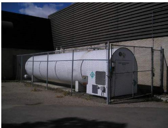
Figure 2.10: Carbon Dioxide Storage Tank
