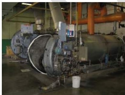
Photo 2.6: ↑ Natural Gas, Steam Generating Boilers
