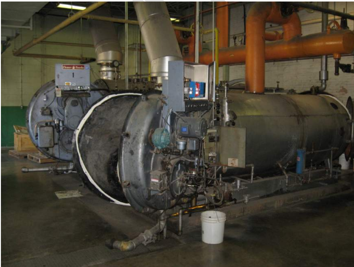
Photo 4.39: ↑ Low Pressure Steam Boilers
