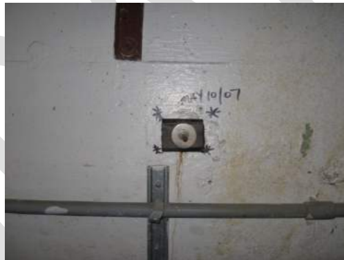
Photo 3.14: ↑ Re-Carbonation Chamber Patch
