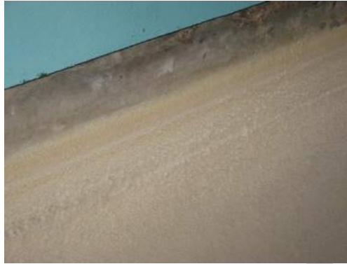
Photo 3.8: ↑ Minor Pitting of Contactor Tank
