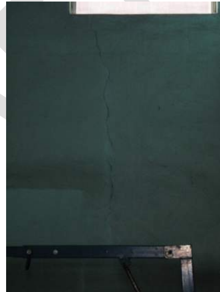
Photo 3.3: ↑ Plant No. 1 Cracking at Contactor Room
