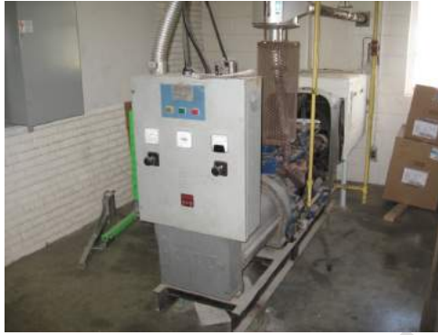
Photo 4.38: ↑ Gas Fired Standby Generator
