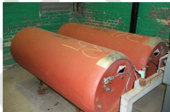
Photo 5.10: ↑ Chlorine Cylinders
