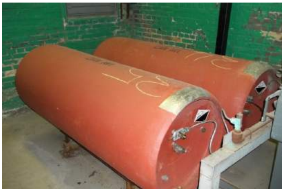
Photo 4.28: ↑ Chlorine Cylinders
