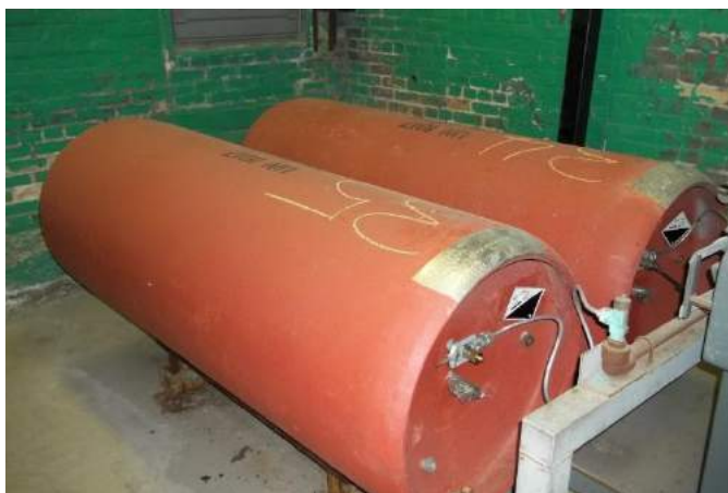
Figure 2.4: 1-Tonne Chlorine Storage Tanks
