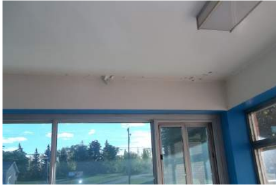
Photo 4.9: ↑ Moisture-Damaged Ceiling
