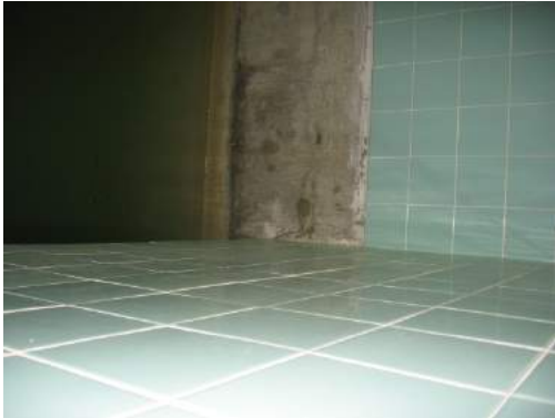
Photo 3.12: ↑ Concrete Cracking at Tile Line
