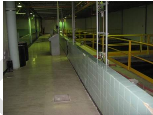
Photo 2.10: ↑ Existing Ceramic Tiled Half Wall
