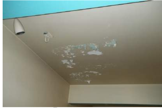
Photo 4.10: ↑ Moisture-Damaged Ceiling
