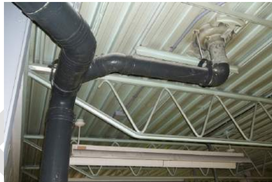
Photo 4.16: ↑ Roof Drainage
