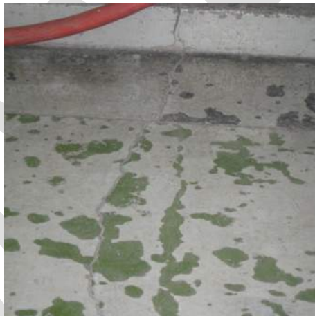
Photo 3.5: ↑ Cracking on Filter Tank Floor
