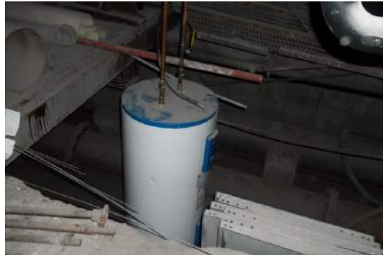
Photo 4.34: ↑ Electric Hot Water Heater Below Staff Lockers
