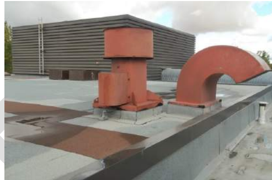
Photo 4.6: ↑ Exhaust Fan and Intake
