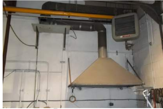
Photo 4.27: ↑ Machine Shop Ventilation
