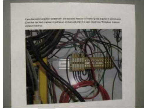
Photo 5.2: ↑ Communications Fault Reset
