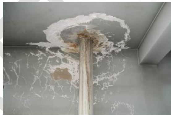
Photo 4.12: ↑ Moisture-Damaged Ceiling
