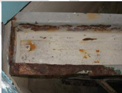
Photo 3.7: ↑ Corrosion of Internal Components of Contactor Tank
