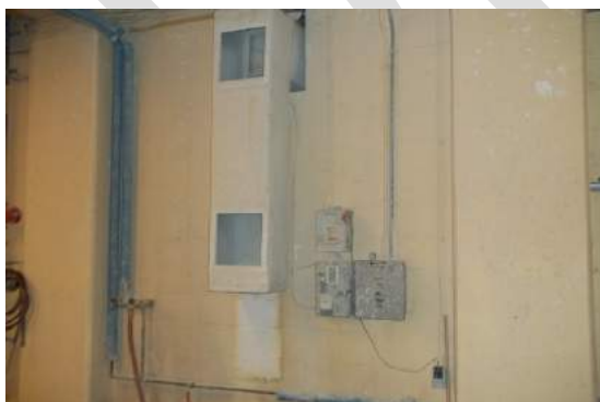
Photo 4.13: ↑ Carbon Monoxide Sensors
