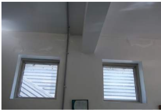
Photo 4.11: ↑ Moisture-Damaged Ceiling
