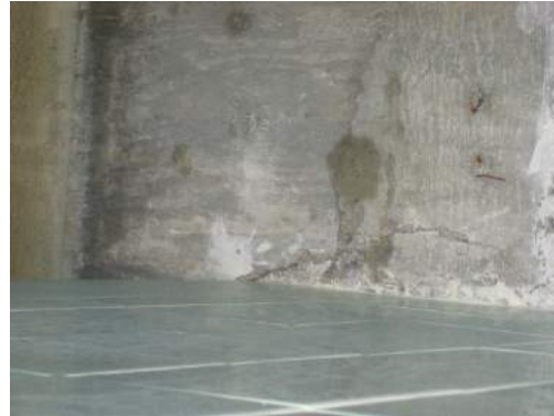
Photo 3.13: ↑ Concrete Cracking at Tile Line
