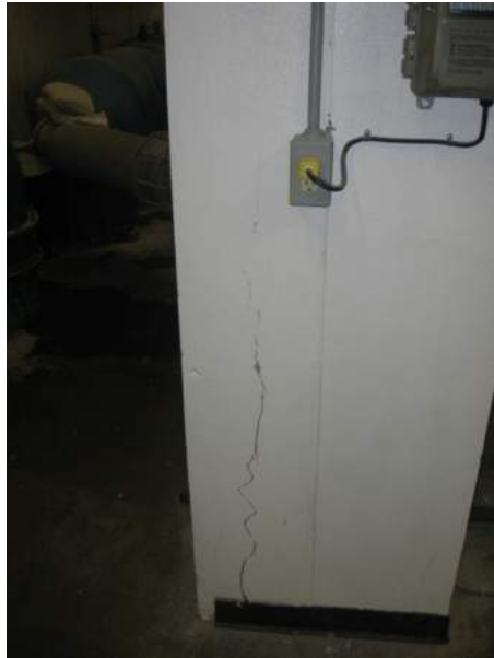
Photo 3.10: ↑ Cracking of Support Columns
