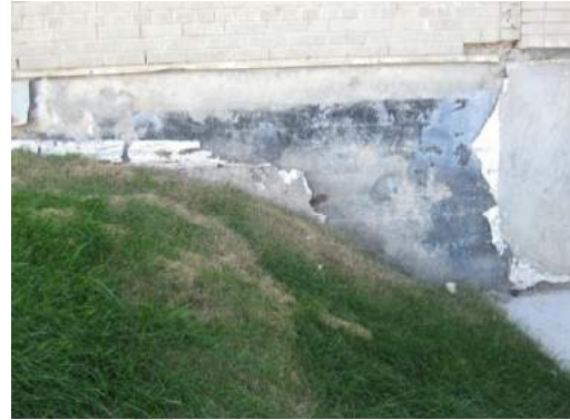
Photo 2.34: ↑ Plant No. 2 Exterior Delamination
