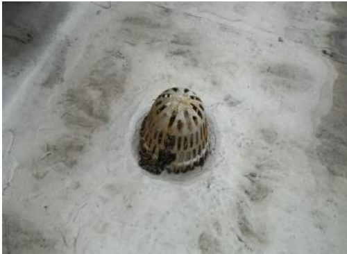
Photo 4.36: ↑ Roof Drains
