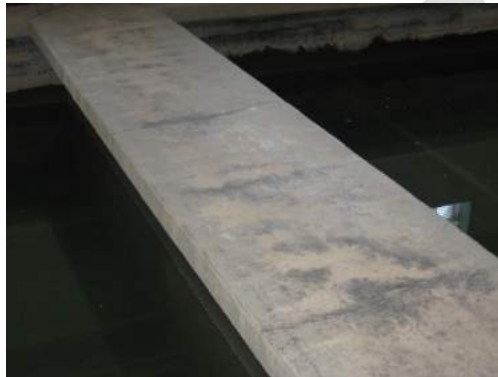
Photo 3.6: ↑ Hairline Cracking in Filter Walkway
