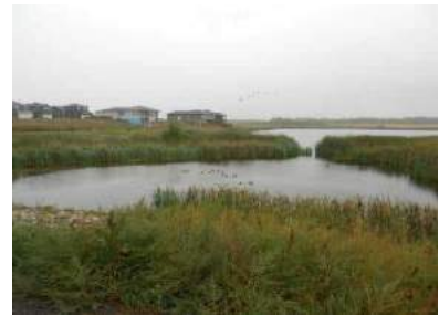
Figure 15: Use of Existing Wetland as a Storm Water Retention Pond
