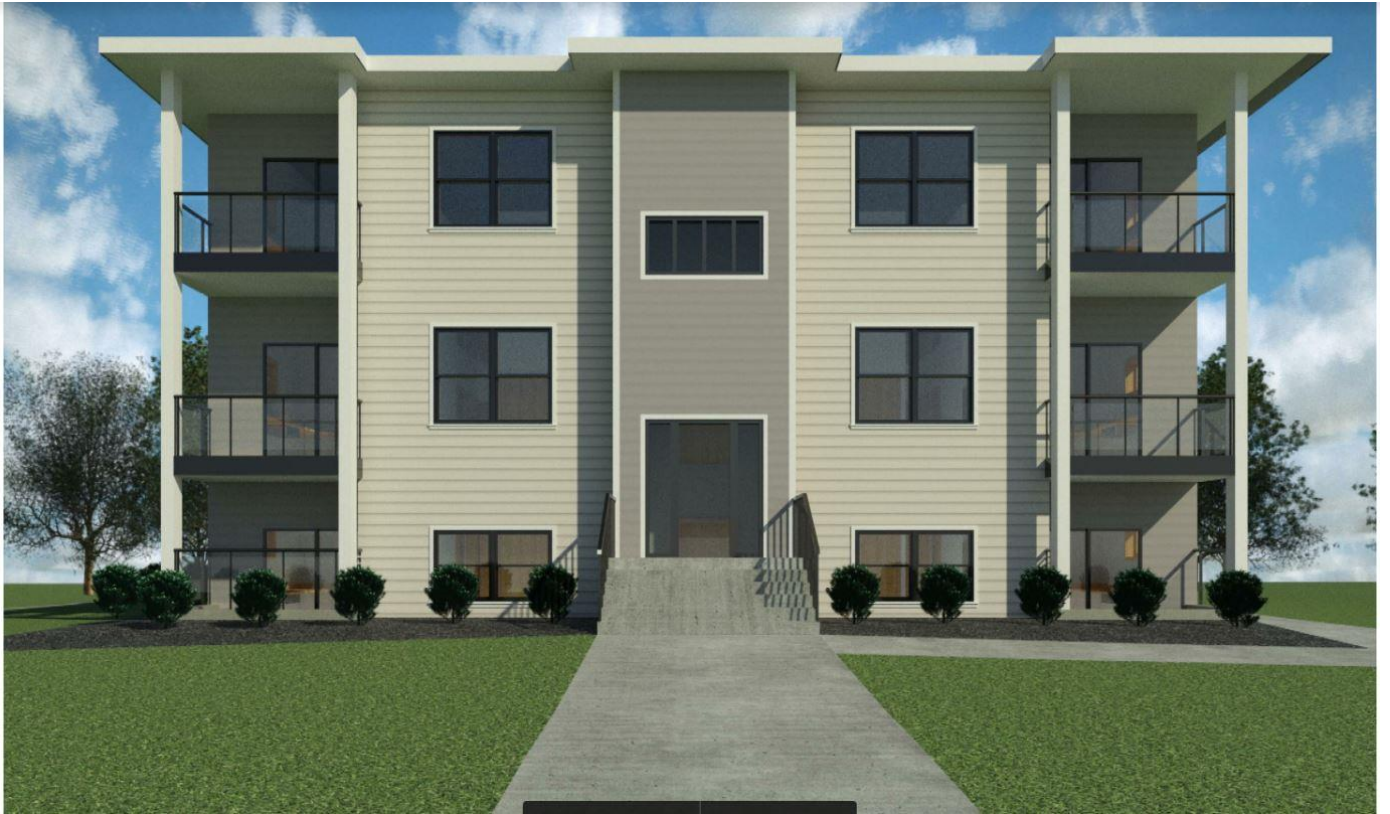
Exterior View from Richmond Avenue
