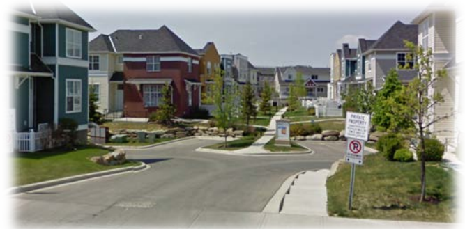
Figure 10: View from street into residential site
