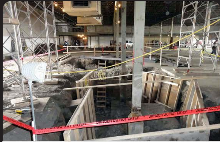
Reinforced footings to strengthen support columns to hold the reinforced roof.
