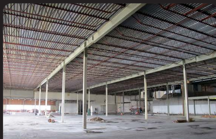
Completed reinforced work on the ceiling.
