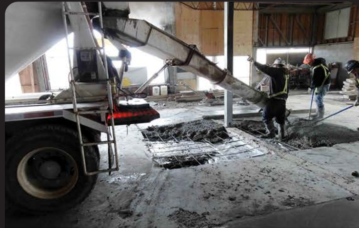
Pouring cement to finish the footings.
