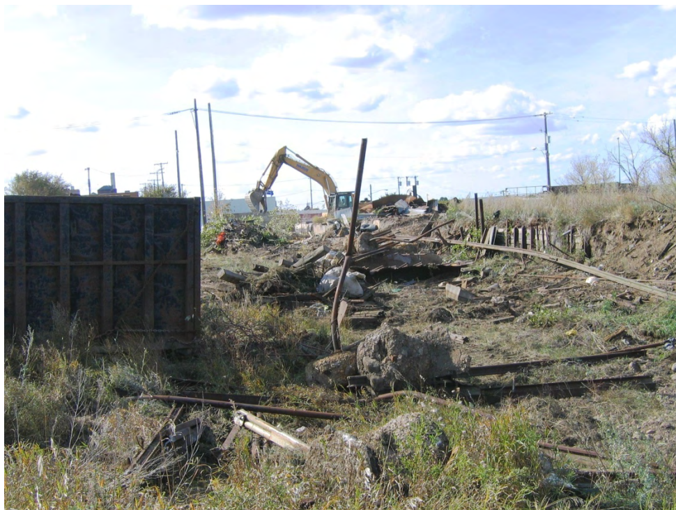
Photograph 1. Clearing site debris. Photograph facing west. (September 2008)
