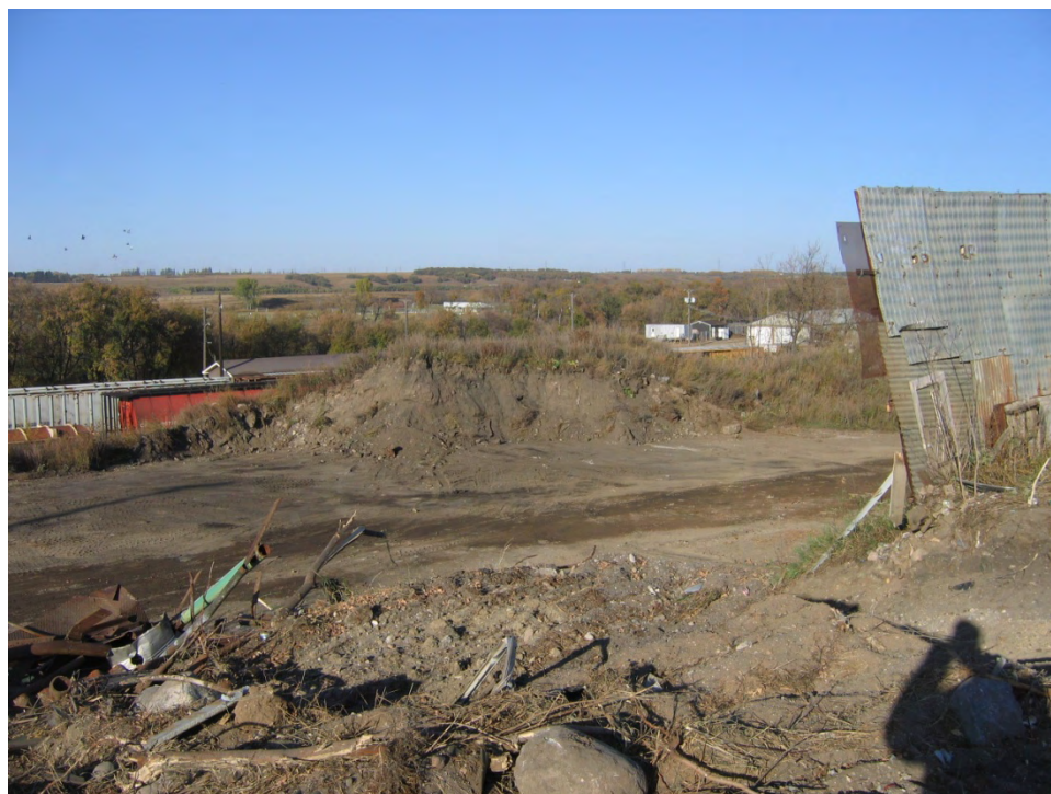
Photograph 4. Moving soil stockpile north of Pacific Avenue. Photograph facing northeast. (October 2008)
