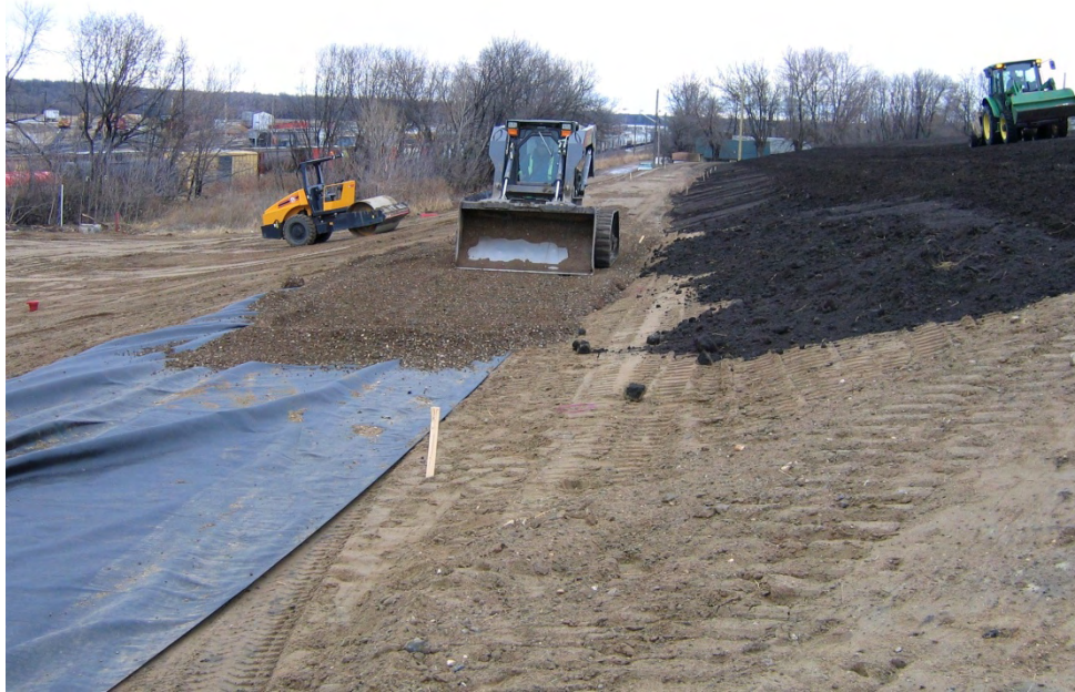
Photograph 15. Placement of walking path base material along north side of engineered cap. Photograph facing east. (November 2008)
