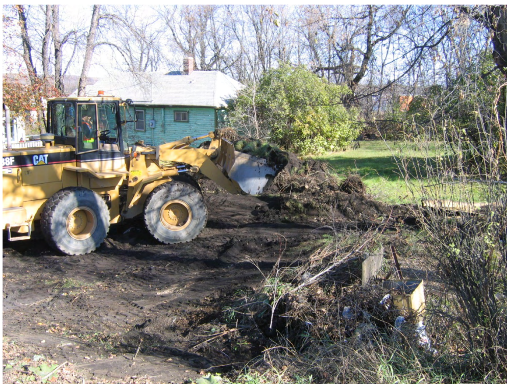
Photograph 8. Residential surface soil excavation. Photograph facing northeast. (October 2008)
