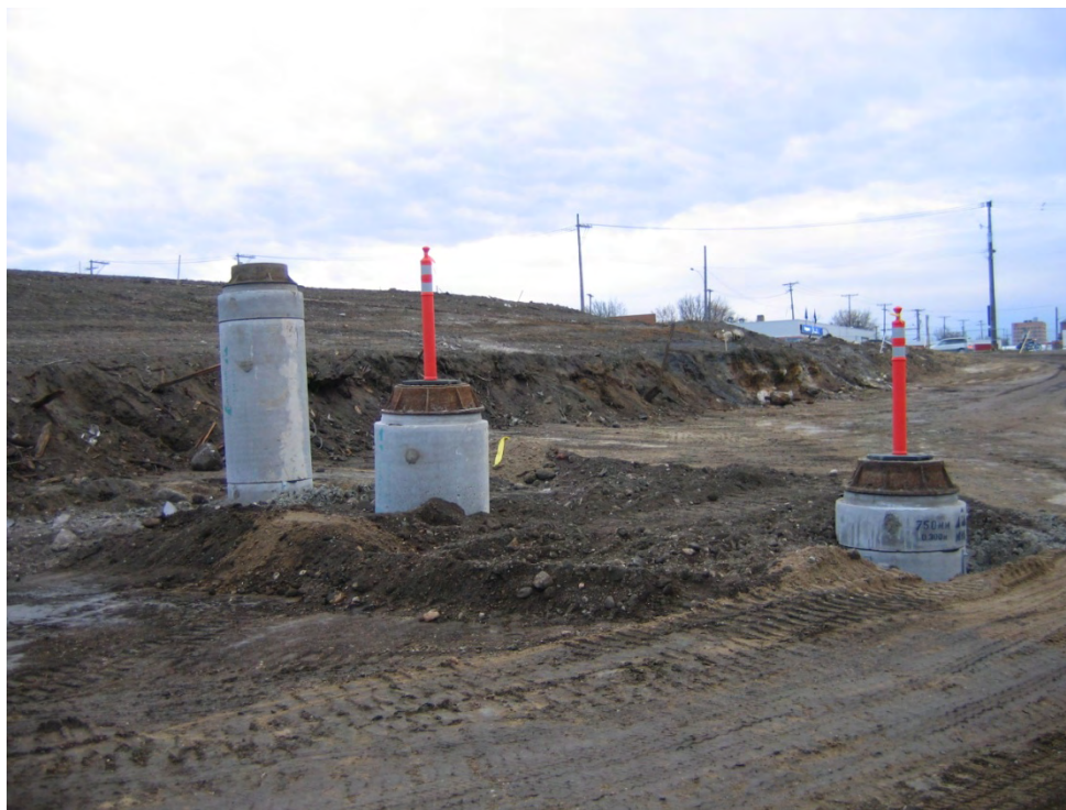
Photograph 13. Adjustment of manhole elevations on Pacific Avenue. Photograph facing west. (October 2008)
