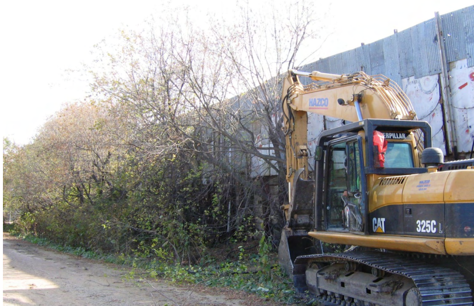
Photograph 2. Clearing trees north of scrap yard fence. Photograph facing southeast (September 2008)
