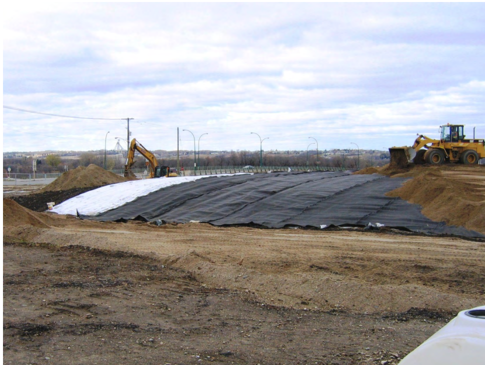
Photograph 11. Installation of GCL (white) and geocomposite drainage layer (black) over impacted soil. Photograph facing north. (October 2008)
