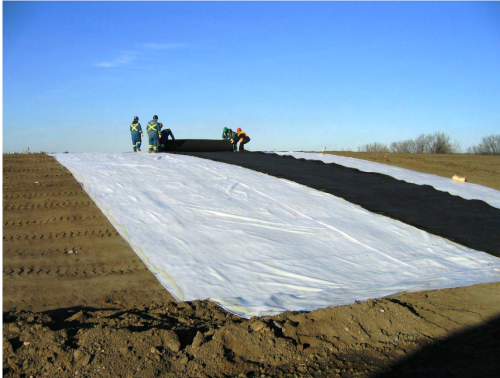
Photograph 11. Installation of GCL (white) and geocomposite drainage layer (black) over impacted soil. Photograph facing north. (October 2008)
