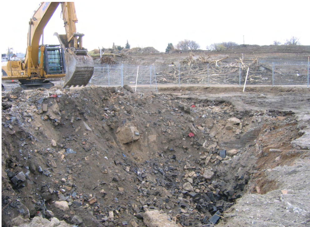
Photograph 9. Subsurface soil excavation north of Pacific Avenue. Photograph facing south. (October 2008)
