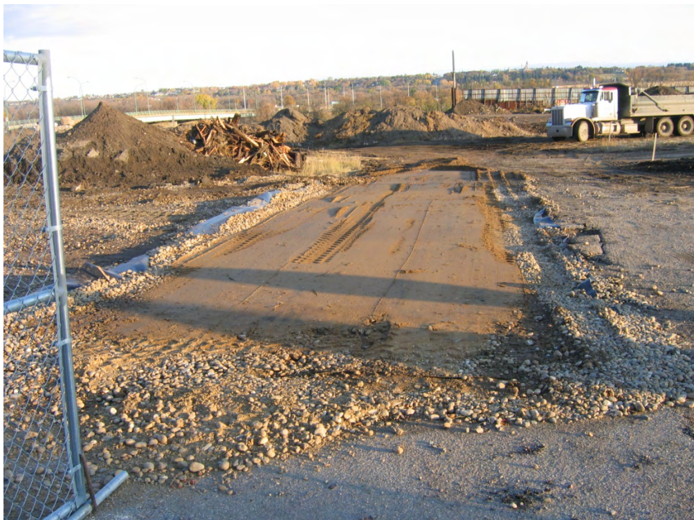
Photograph 6. Decontamination pad for vehicles. Photograph facing north. (October 2008)
