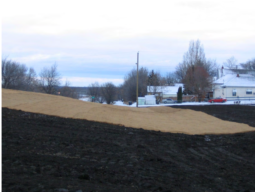
Photograph 15. Placement of walking path base material along north side of engineered cap. Photograph facing east. (November 2008)
