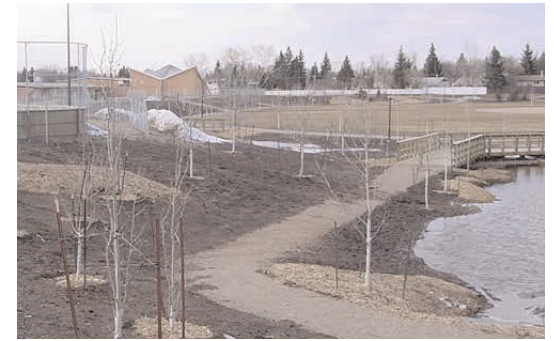
This greenspace in Regina provides an example of an innovative approach to integrating greenspace amenities with stormwater management practices.
